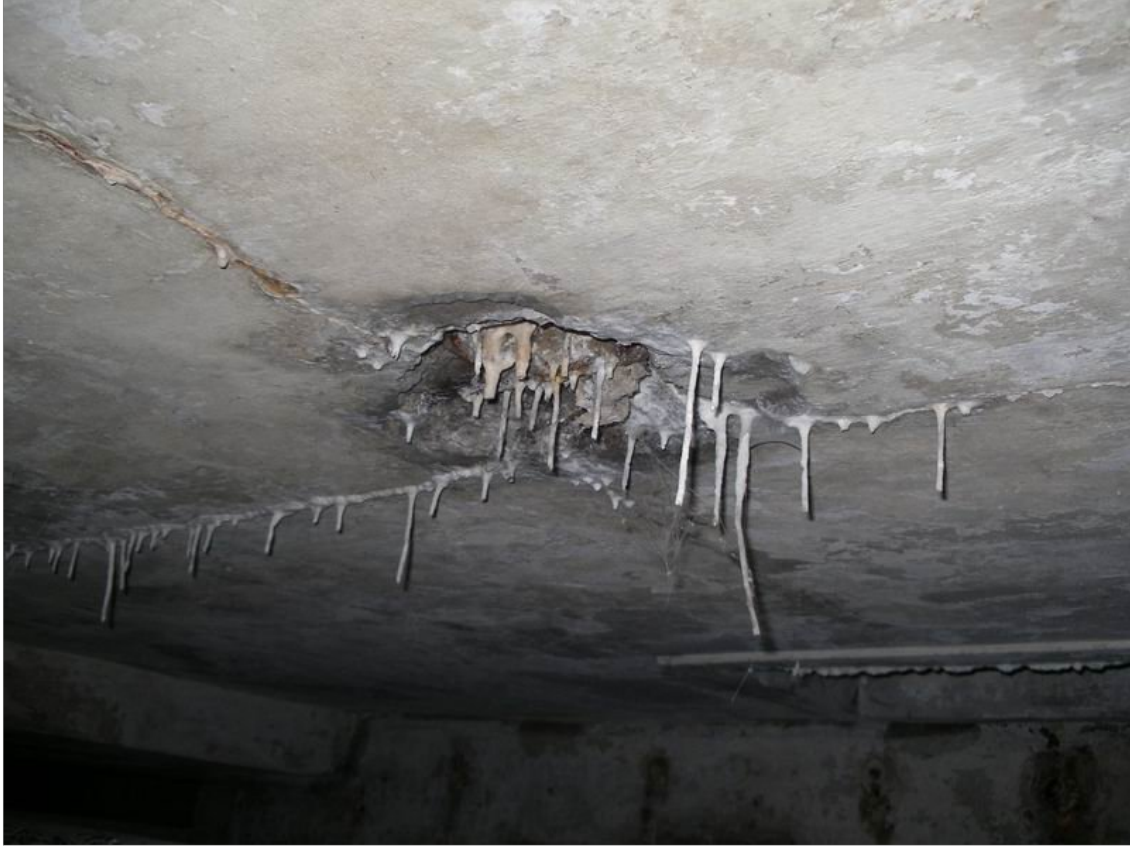
Belgrade, Monument in the honour of Belgrade defenders 1914-1918: salting out of construction material
