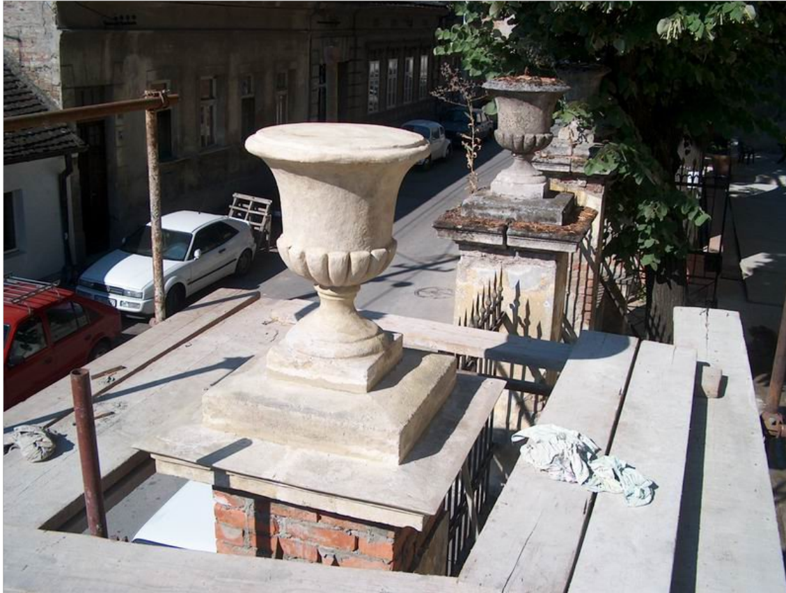
Zemun, Saint Father Nikolaj Temple: stone vase and capital after cleaning, restoration and conservation and vase and capitals which were not treated (in the background)
