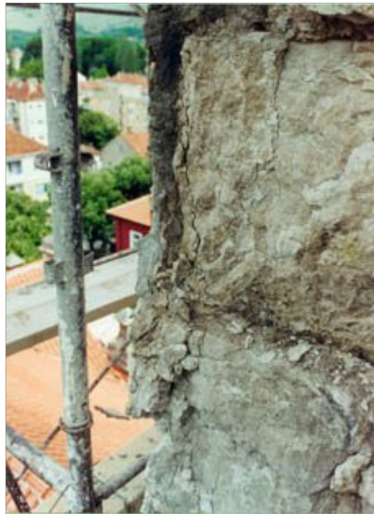
Trebinje, Serbian Orthodox Temple (balcony, South and North facade): damages on the stone
